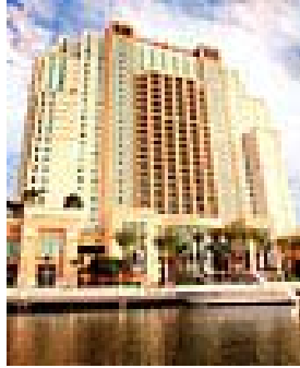
Marriott Tampa Waterside
